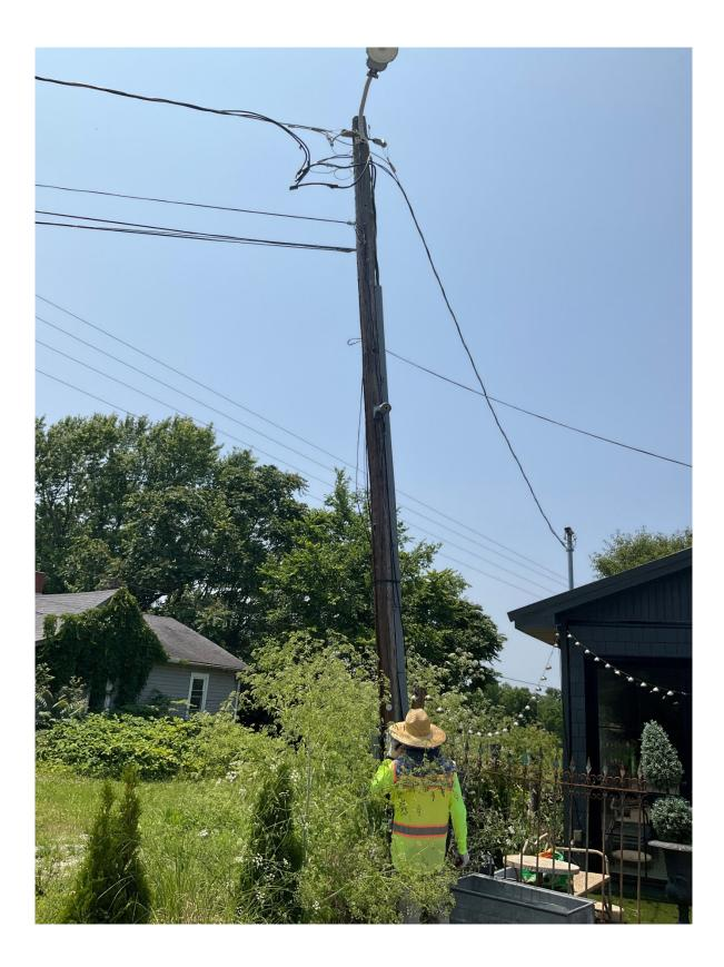
Low Height at Midspan Figure 6 – Communications attachment appears to not be pulled to proper tension causing low midspan height.
