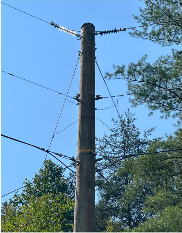
Example #2 of Yellow Communication Band at transition point between communication and power space.
