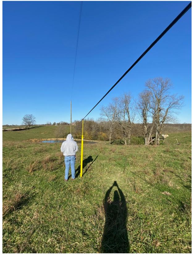
Unbalanced Line Tension Figure 7 – Unguyed angle attachment causing pole to lean in direction of unbalanced load. This can be dangerous for
